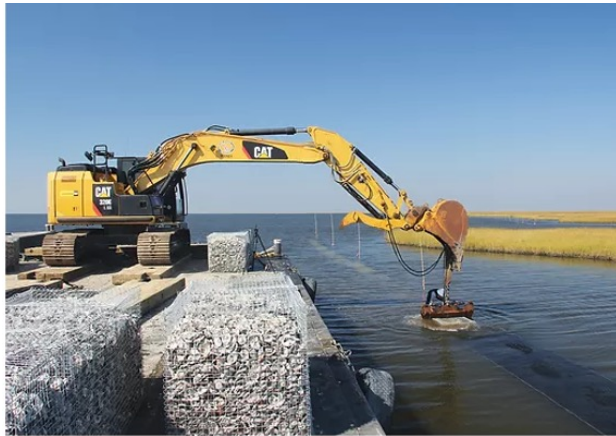
7 Deploying cages of oyster shell for restoration in Louisiana (CRCL)
